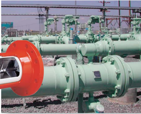
Smith 6" MV Series Turbine Meters installed at a pipeline terminal facility.
